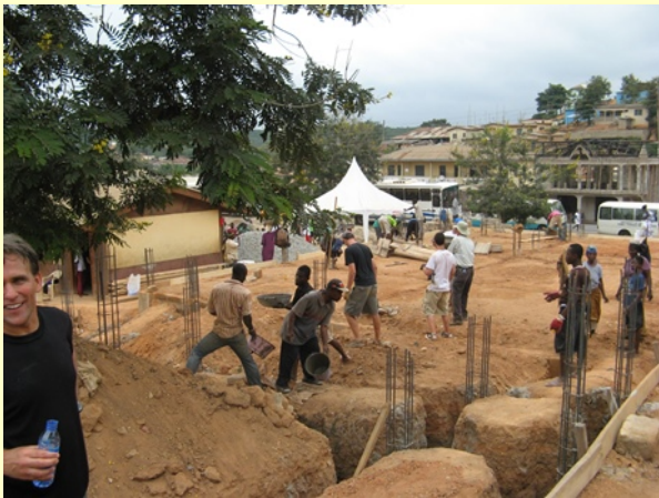
Construction in summer 2012. YASC works with community on the foundation of the ICTC
