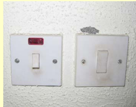
Button on the left is the water heater switch
