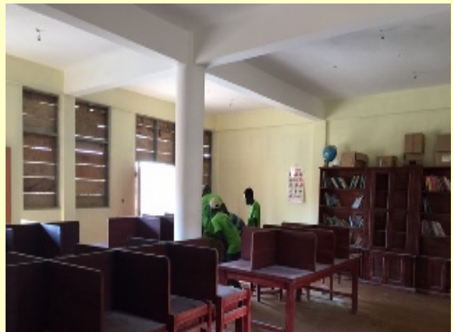
The inside of the ICTC Library (nearly finished) taken this past fall.
